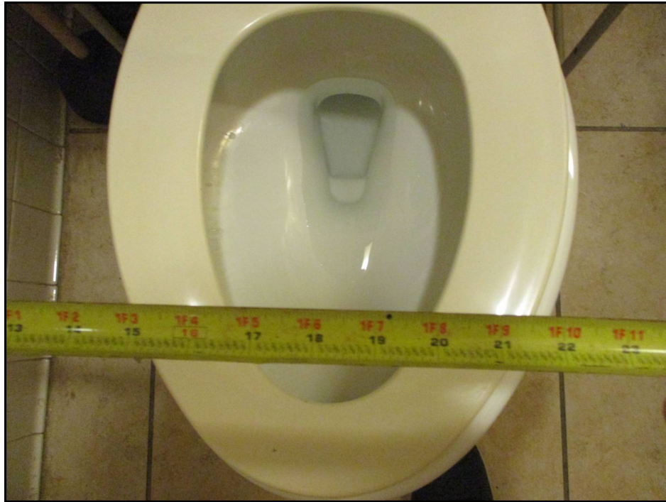
29: Compliant Handicapped Dwelling Unit Bathroom Toilet Centerline Spacing to Adjacent Wall
