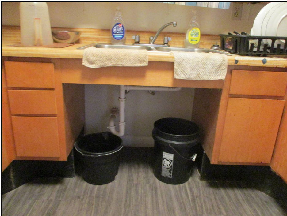
46: Non-Compliant Handicapped Dwelling Unit Kitchen Roll-Under Sink Missing Scald/Abrasion Protection and Levered Hardware (Critical Repair)
