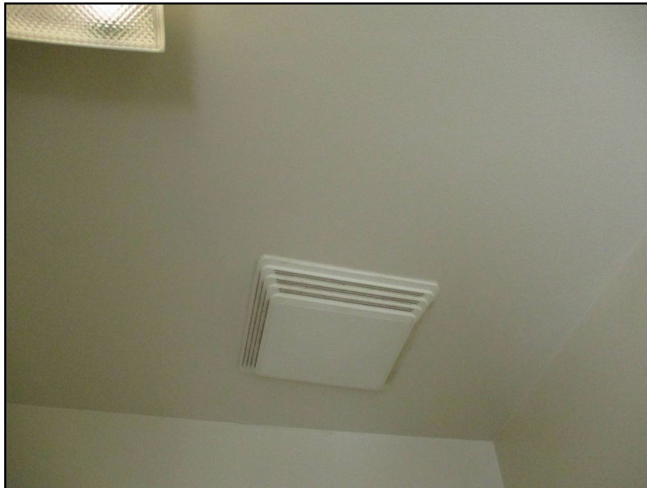
8: Common Area Restroom Exhaust Fan
