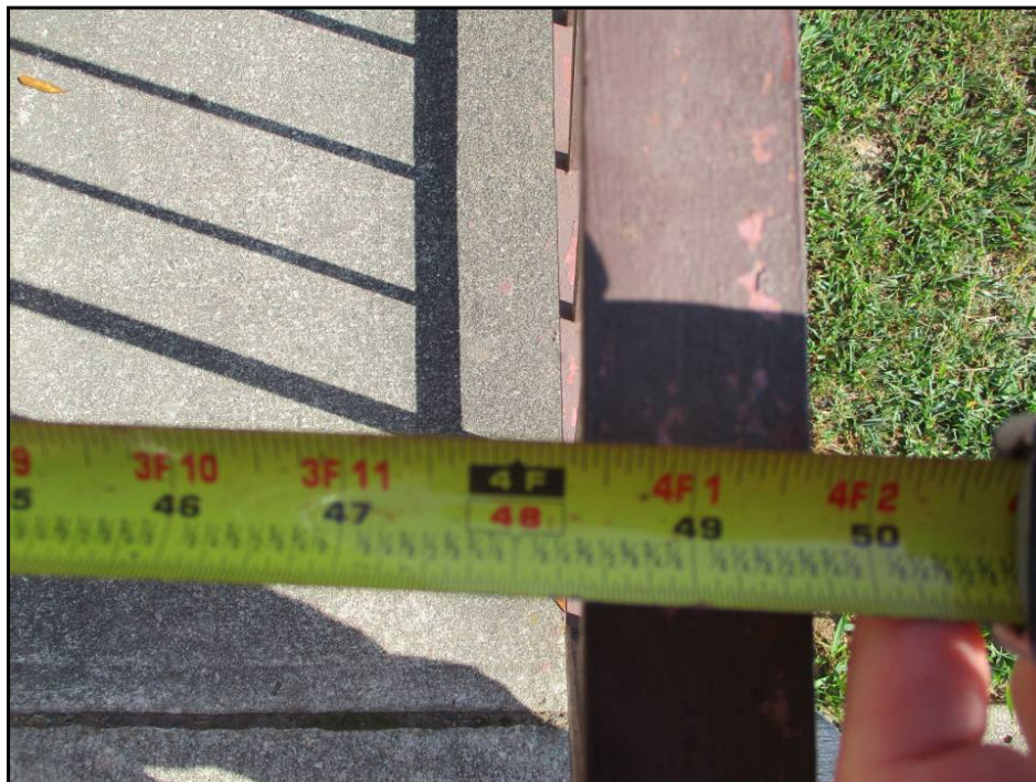
2: Compliant Exterior Accessible Route Clear Width
