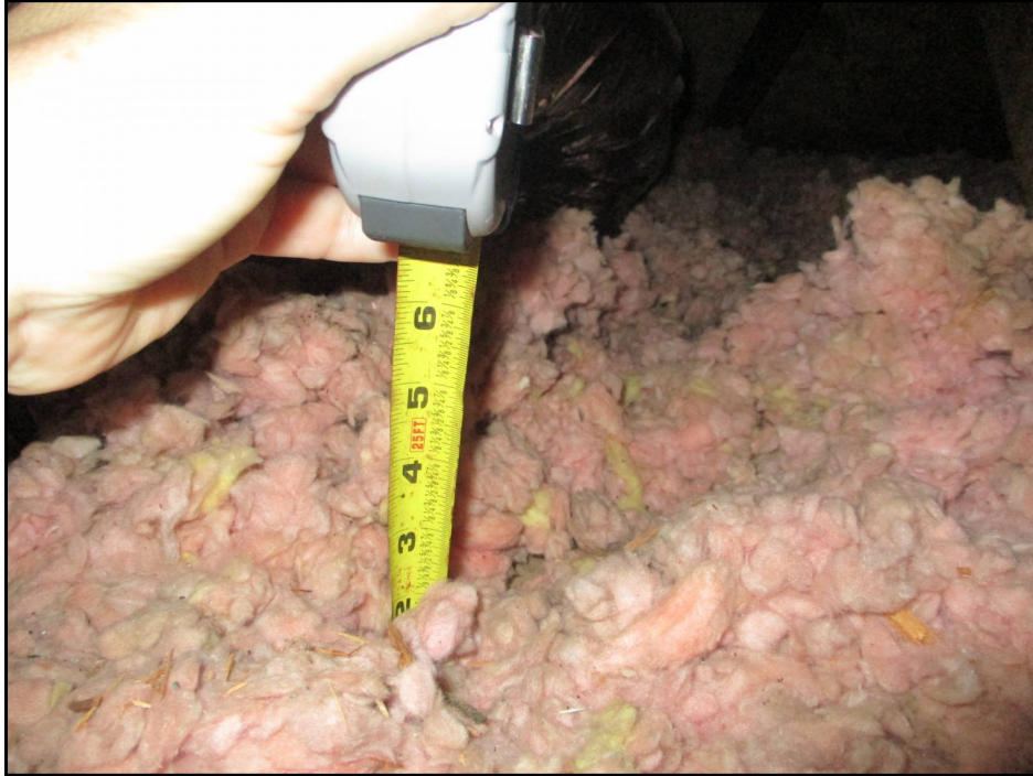
5: Install Code Compliant Attic Insulation- (Non-Critical Repair)
