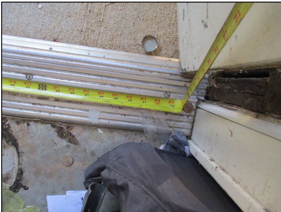
20: Compliant Handicapped Dwelling Unit Exterior Storage Room Door Clear Opening Width
