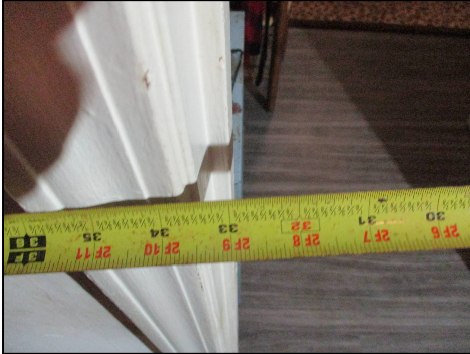
25: Compliant Handicapped Dwelling Unit Interior Door Clear Opening Width
