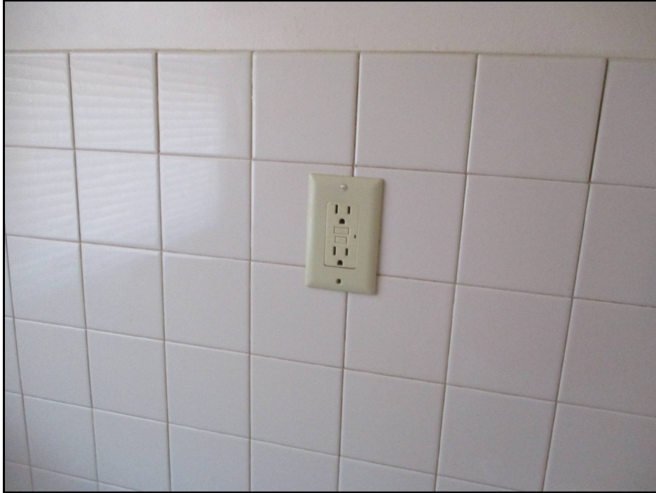
21: Dwelling Unit Bathroom Outlet with GFCI Protection
