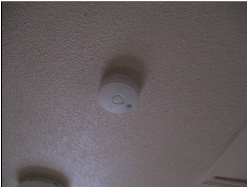
26: Tamper Proof Battery-Powered Smoke Detectors in Dwelling Unit Sleeping Areas
