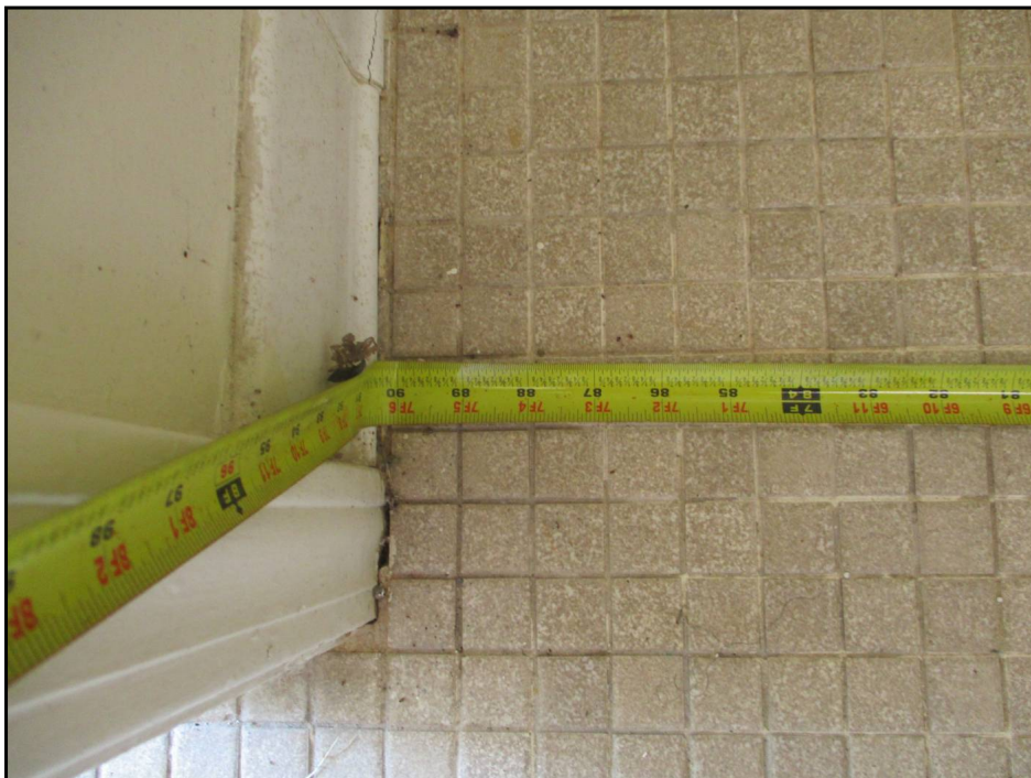
10: Compliant Common Area Restroom Clear Floor Space
