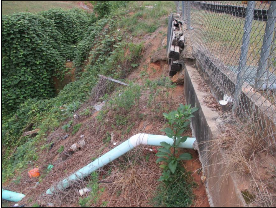
1: Correct Erosion Issues and Repair Retaining Walls and Fencing (Critical Repair)
