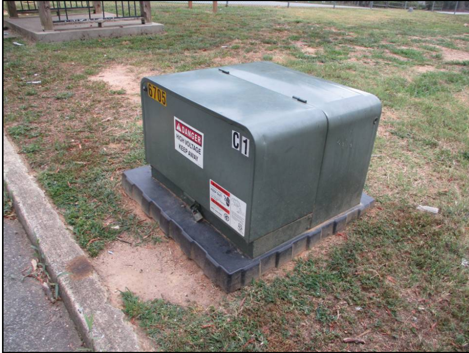
15: Pad Mounted Electrical Transformer
