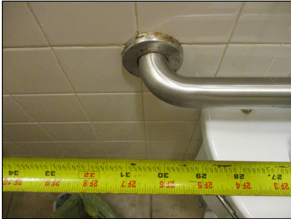
49: Non-Compliant Handicapped Dwelling Unit Bathroom Rear Toilet Grab Bar Length (Critical Repair)
