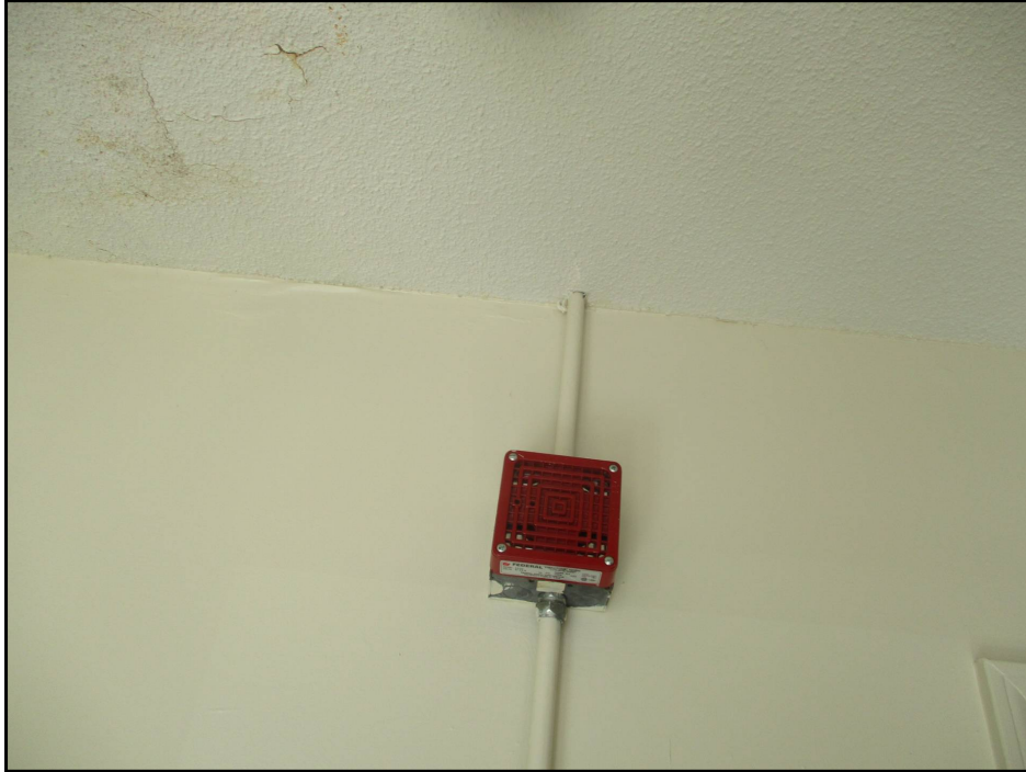
29: Common Area Fire Alarm System Audio Alarm Device
