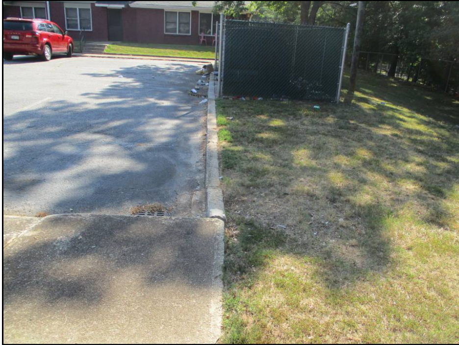
35: Non-Compliant Site Amenity (Dumpster) Missing Accessible Route (Critical Repair)
