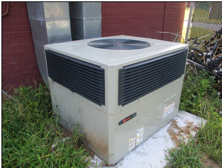
4: Common Area Packaged HVAC Unit
