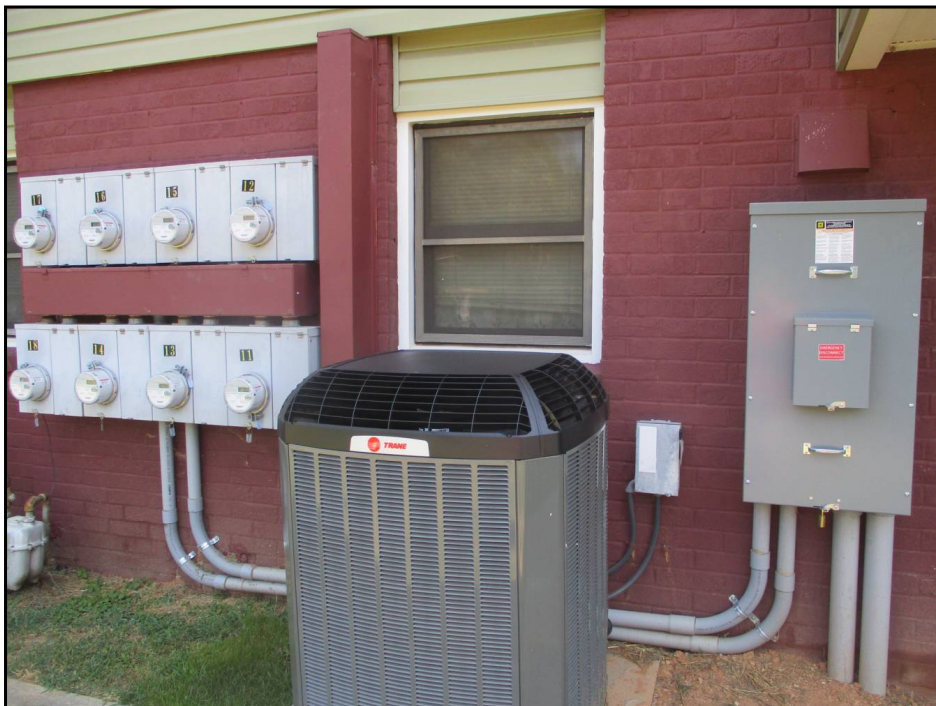
16: Apartment Building Electrical Service and Meter Bank
