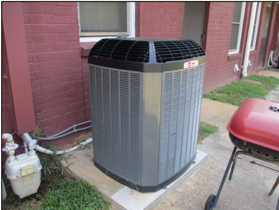
10: Dwelling Unit Exterior Pad Mounted Condensing Unit
