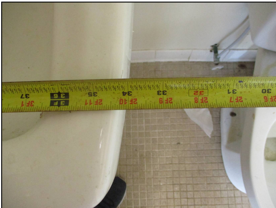
14: Compliant Common Area Restroom Toilet Clear Floor Space
