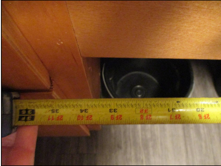
23: Compliant Handicapped Dwelling Unit Kitchen Roll-Under Sink Clear Width
