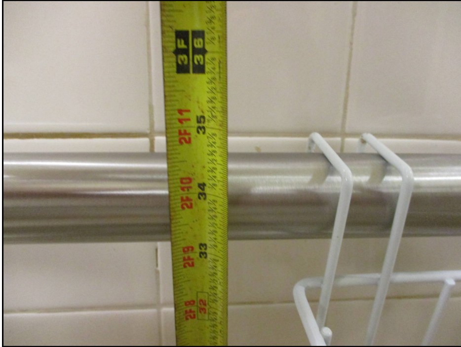
31: Compliant Handicapped Dwelling Unit Bathroom Toilet Grab Bar Height
