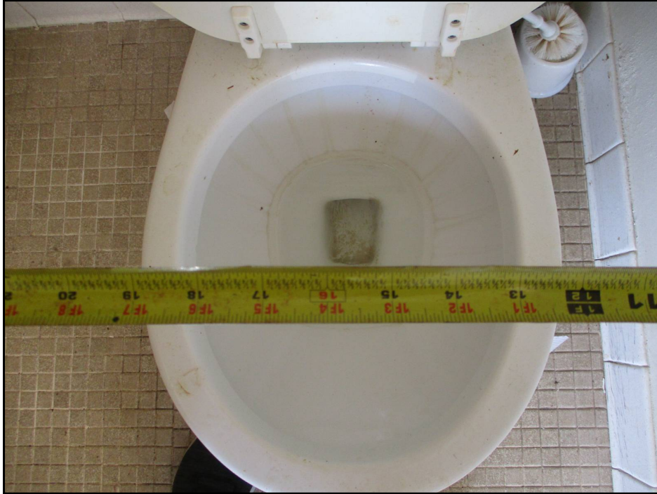
13: Compliant Common Area Restroom Toilet Centerline Spacing to Adjacent Wall
