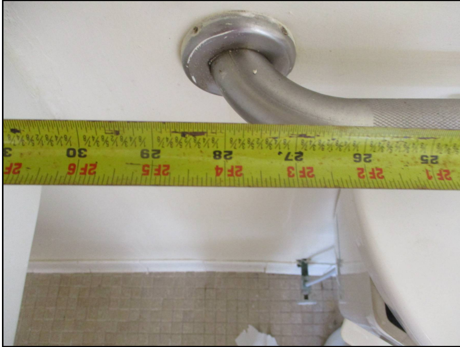
41: Non-Compliant Common Area Restroom Rear Toilet Grab Bar Length (Critical Repair)
