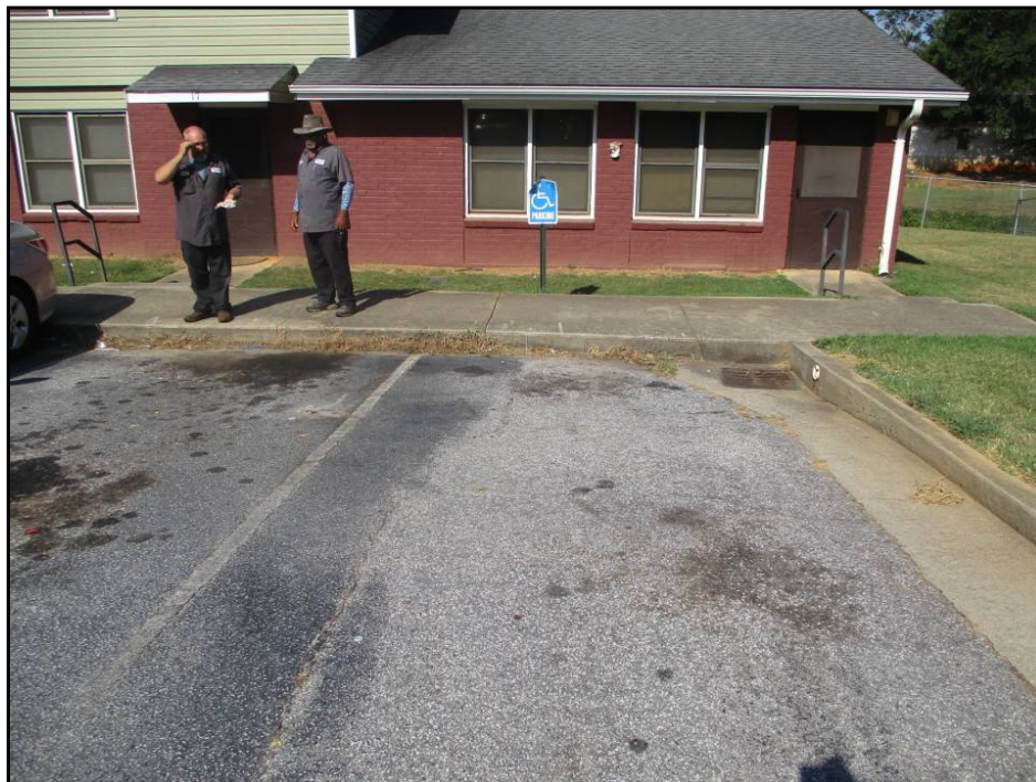
34: Non-Compliant Handicapped Parking Missing Access Aisle, Pavement Markings and Curb Access (Critical Repair)
