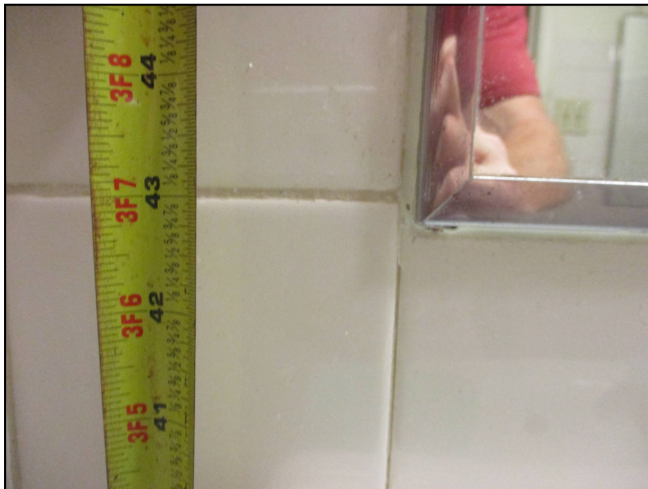
50: Non-Compliant Handicapped Dwelling Unit Bathroom Mirror Height (Critical Repair)
