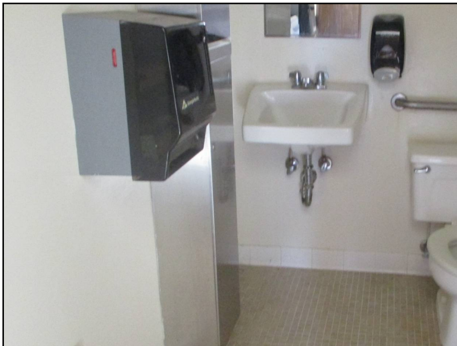
40: Non-Compliant Common Area Restroom Roll-Under Sink Missing Scald/Abrasion Protection (Critical Repair)
