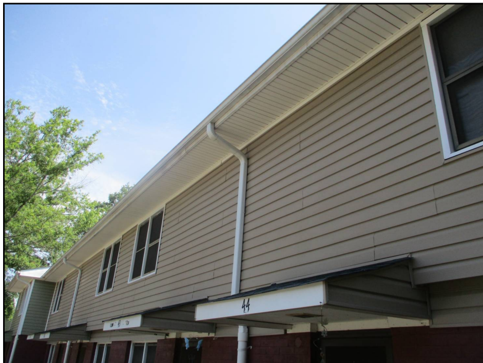
22: Apartment Building- Vinyl Siding, Soffits/Fascia and Gutters & Downspouts
