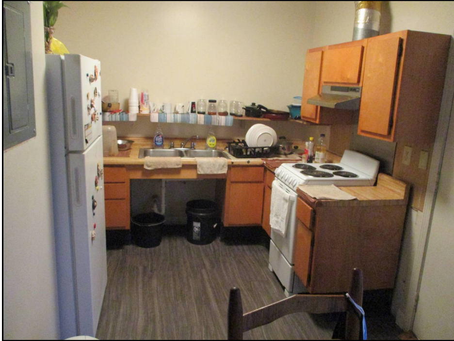
21: Compliant Handicapped Dwelling Unit Kitchen Sink with Roll-Under Access
