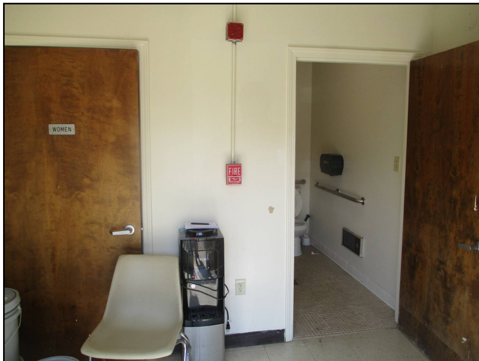
8: Compliant Common Area Restroom Doors with Levered Hardware
