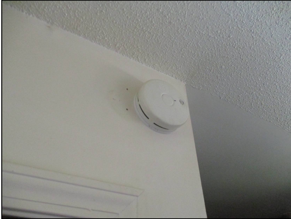
25: Tamper Proof Battery-Powered Smoke Detectors Outside of Dwelling Unit Sleeping Areas
