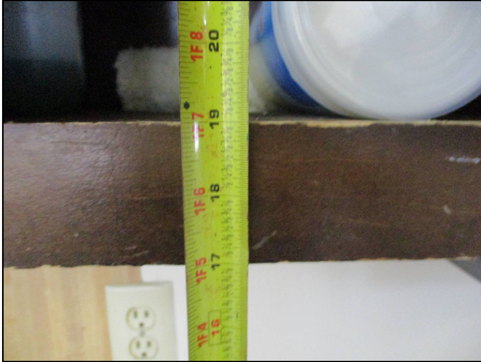
39: Non-Compliant Common Area Kitchen Wall Cabinet Height (Critical Repair)
