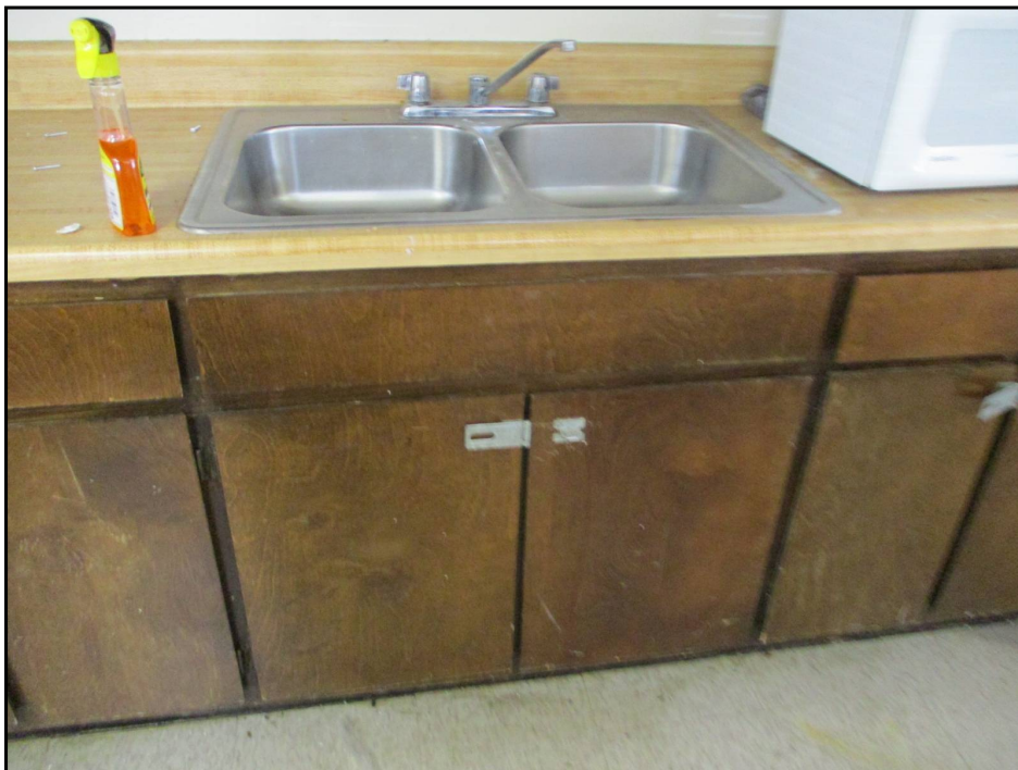
38: Non-Compliant Common Area Kitchen Sink Missing Roll-Under Access (Critical Repair)
