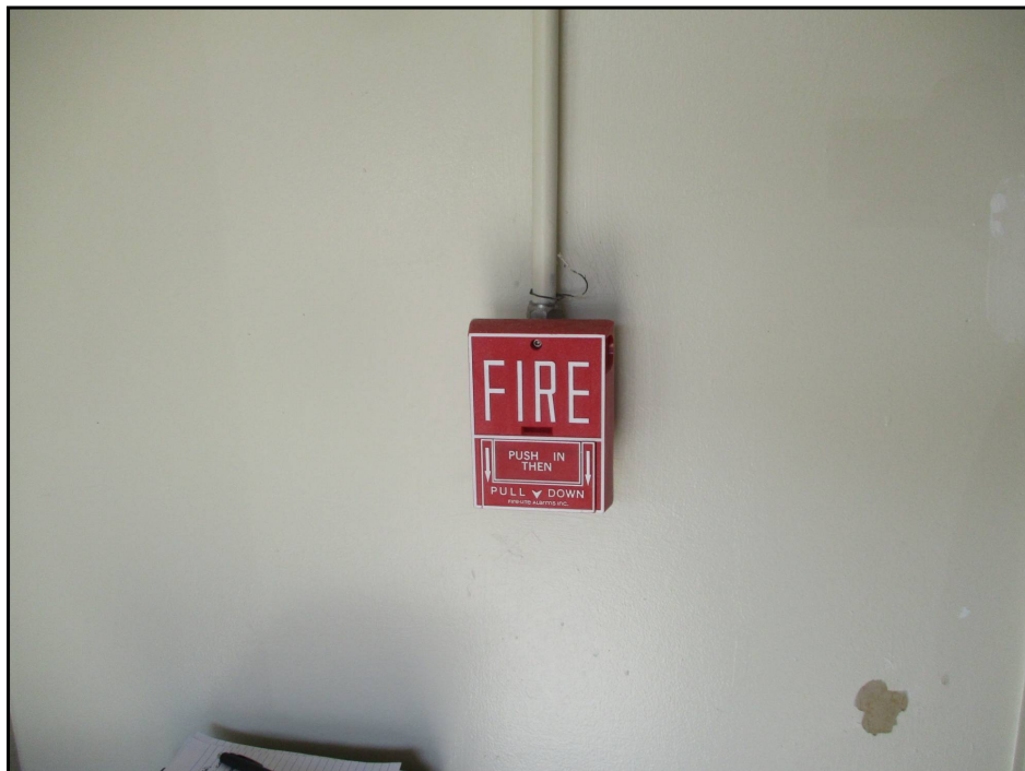
28: Common Area Fire Alarm System Pull Station
