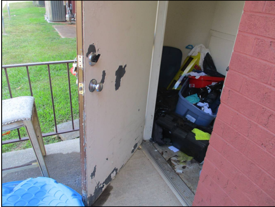
43: Non-Compliant Handicapped Dwelling Unit Exterior Storage Room Door Missing Levered Hardware (Critical Repair)
