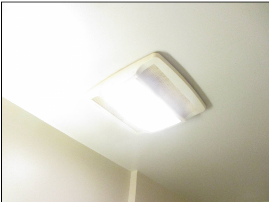
14: Dwelling Unit Bathroom Exhaust Fan
