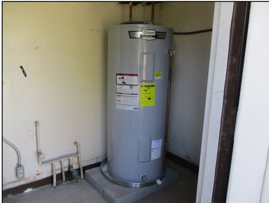
2: Common Area Electric Water Heater
