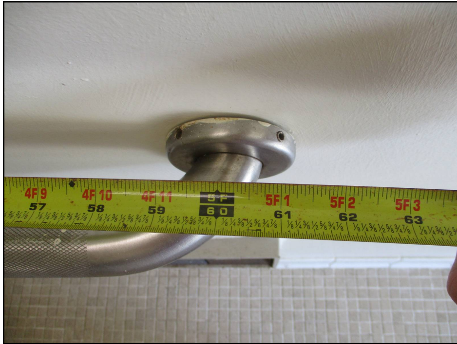
15: Compliant Common Area Restroom Toilet Side Grab Bar Length
