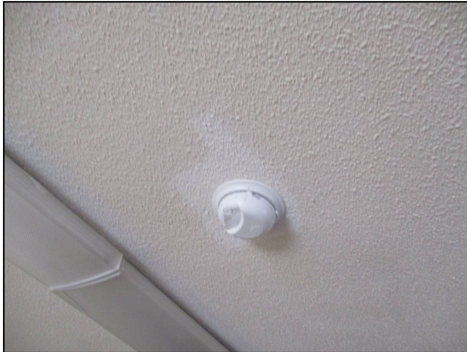
23: Common Area Hard-Wired Smoke Detector
