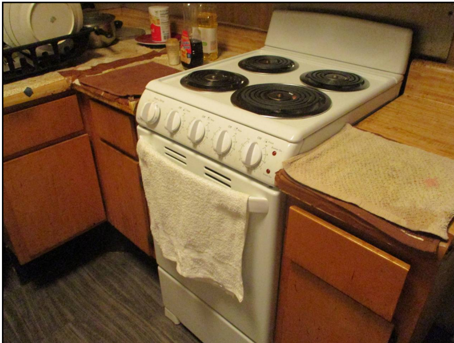
24: Compliant Handicapped Dwelling Unit Kitchen Front-Control Range
