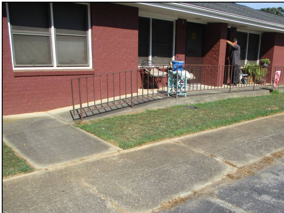
16: Compliant Handicapped Dwelling Unit Entry Door on Accessible Route
