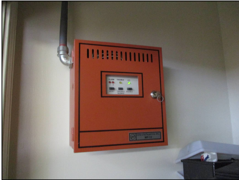
27: Common Area Fire Alarm System Control Panel
