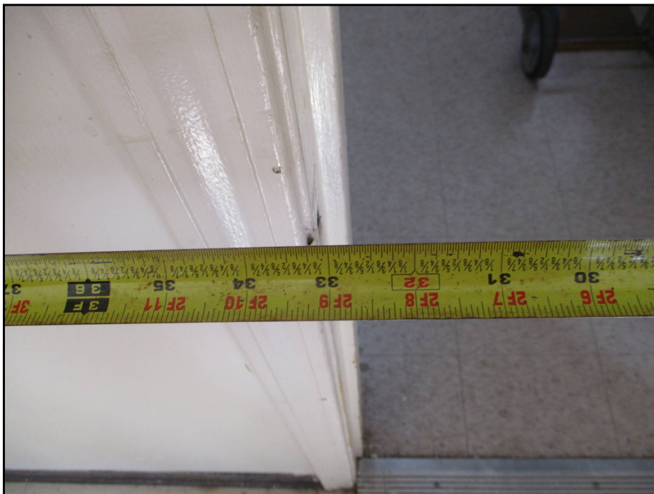
6: Compliant Community Room Entry Door Clear Opening Width
