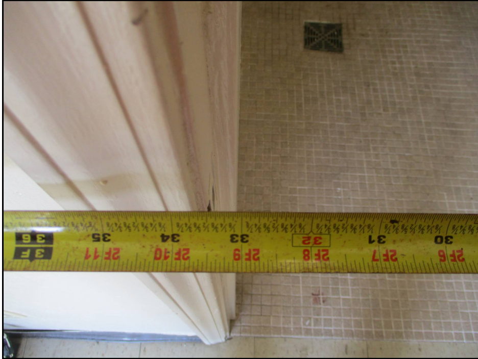
9: Compliant Common Area Restroom Doors Clear Opening Width
