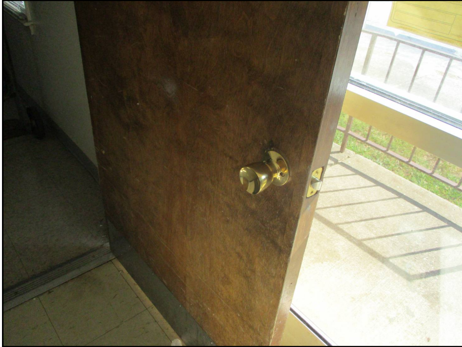
37: Non-Compliant Community Room Door Missing Levered Hardware (Critical Repair)
