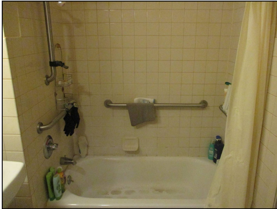
33: Compliant Handicapped Dwelling Unit Bathroom Tub/Shower Grab Bar, Levered Control Hardware, 60-Inch Showerhead Hose
