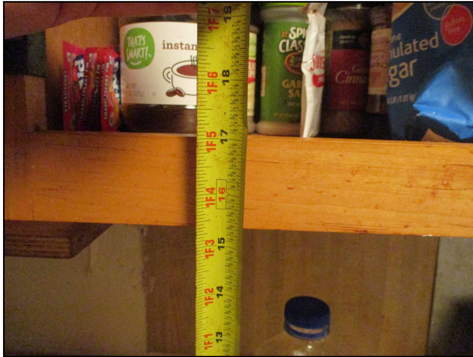
47: Non-Compliant Handicapped Dwelling Unit Kitchen Wall Cabinet Height (Critical Repair)
