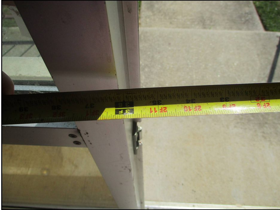
5: Compliant Common Area Entry Door Clear Opening Width
