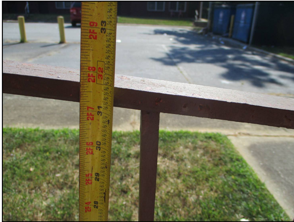
3: Compliant Exterior Ramp Handrail Height
