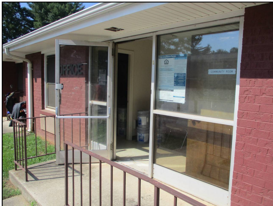
4: Compliant Common Area Entry Door with Egress Hardware
