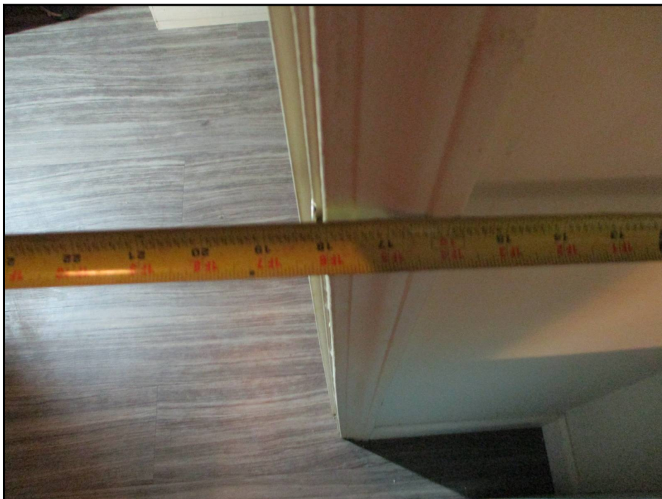
26: Compliant Handicapped Dwelling Unit Interior Door 18-Inches at Pull Side
