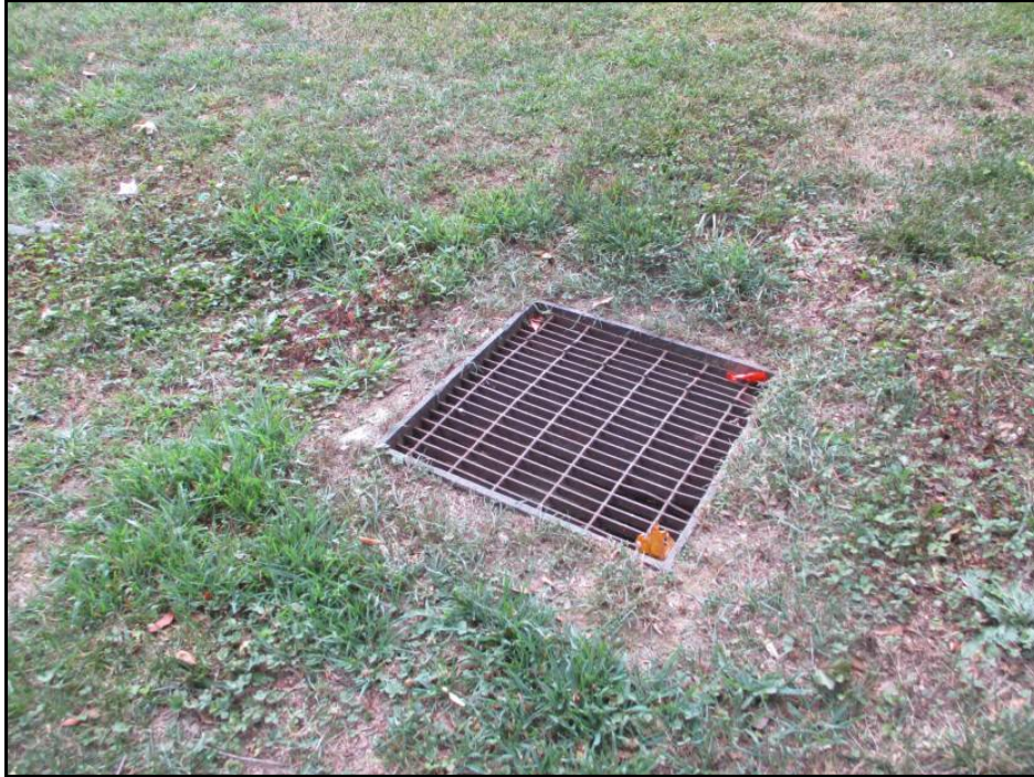
13: Storm Drainage Yard Inlet
