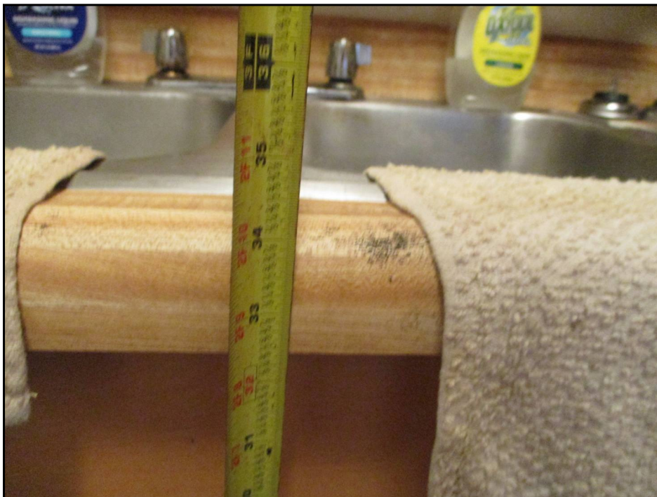
22: Compliant Handicapped Dwelling Unit Kitchen Roll-Under Sink Counter Height
