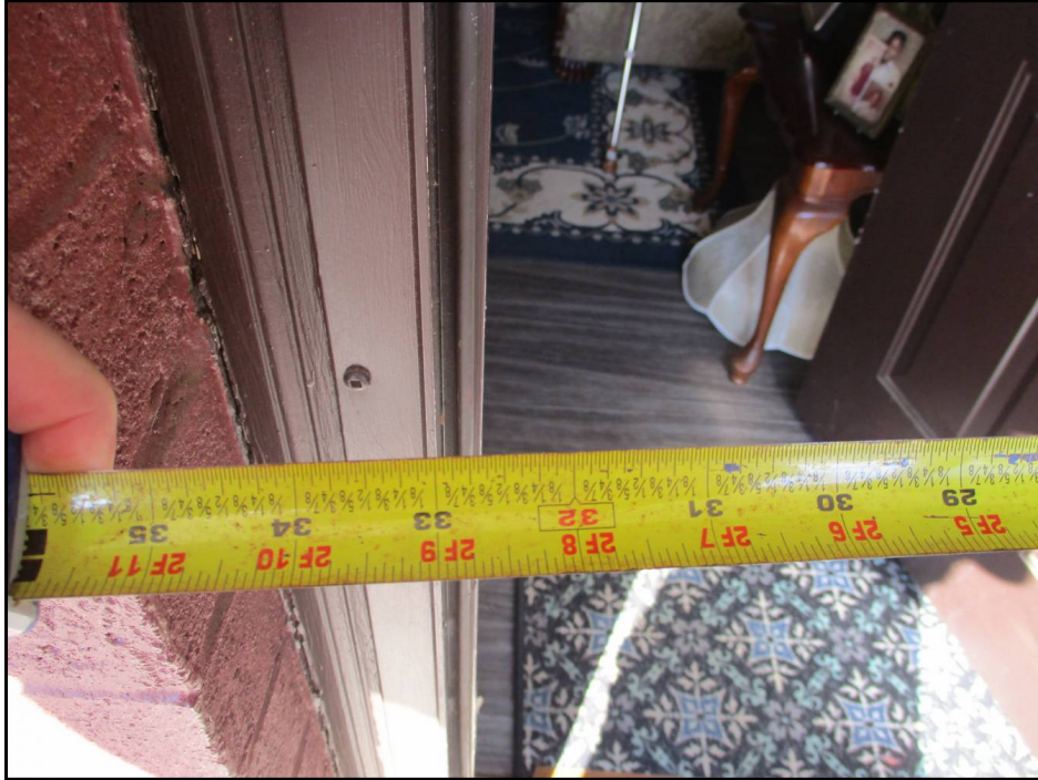
17: Compliant Handicapped Dwelling Unit Entry Door Clear Opening Width
